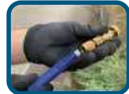
Inserting new gasket
