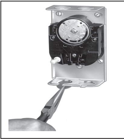
Fig. 5 - Removing slotted knockouts.
